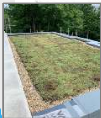
Warm flat green roof assimilating appearance
