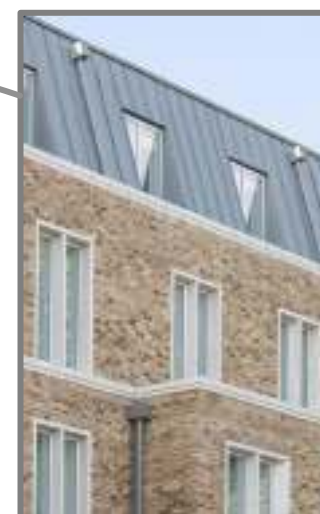
Standing Seam roof enclosure providing an aesthetic screen
